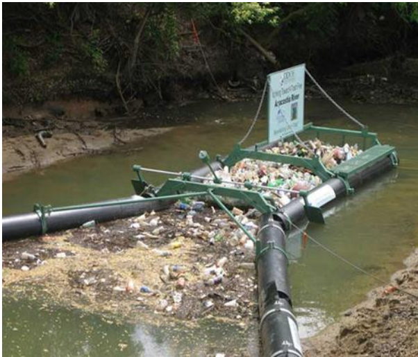
Bandalong Litter Trap in DC ( Stormwater Systems )
