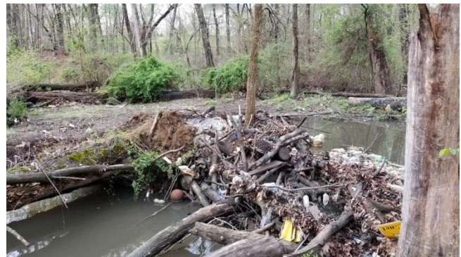
At this Gum Springs dam, the upstream water level was 4 feet higher than downstream ( Betsy Martin )
